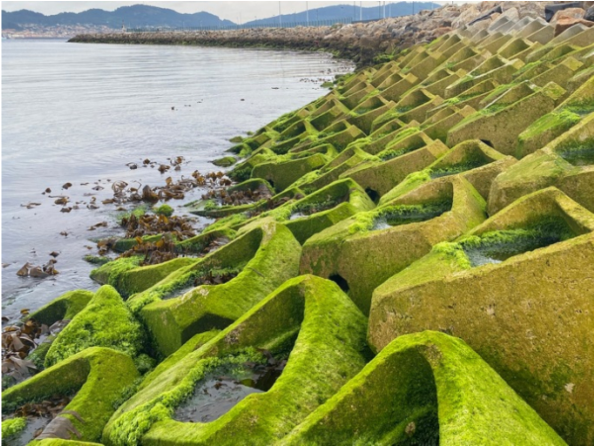
Figure 6: ECONcrete bio-enhancing coastal protection units used in the Living Ports Project at the Port of Vigo [14]
