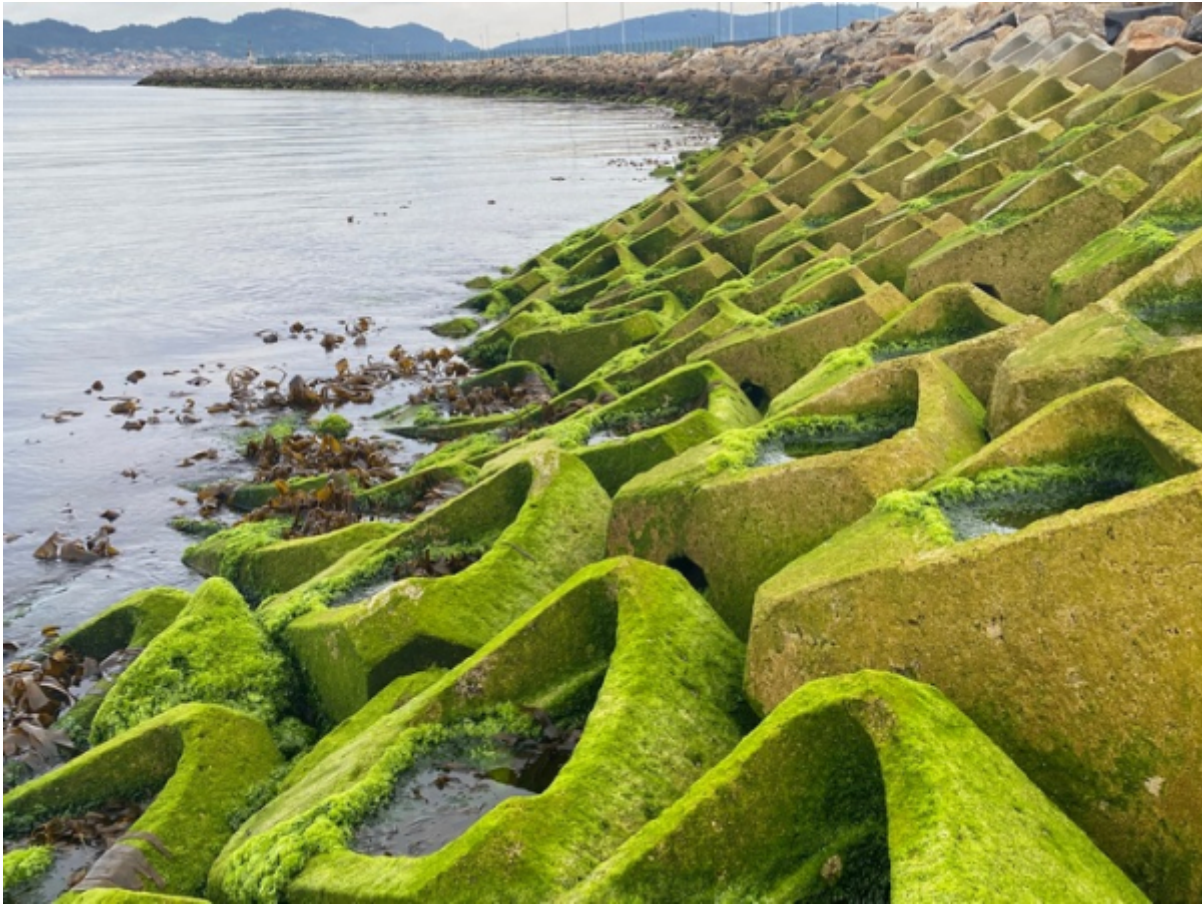
Figure 2: ECONcrete bio-enhancing coastal protection units used in the Living Ports Project at the Port of Vigo [16]
